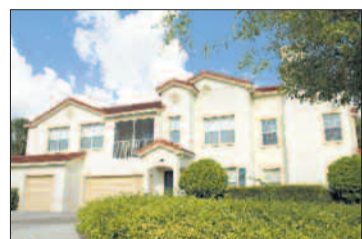
2. ESTATES AT STUART CONDOMINIUM
